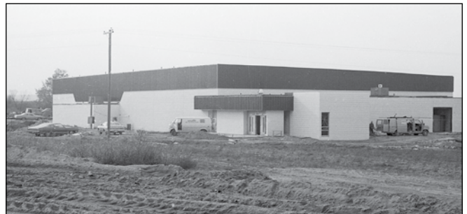
Scugog's new arena under construction in 1976.
