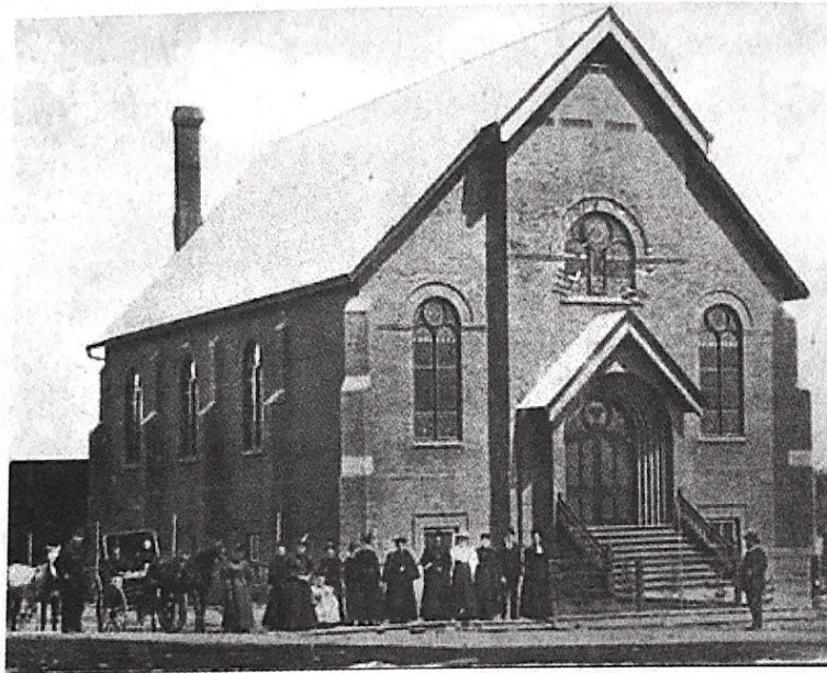
Greenbank Methodist Church, 1909
