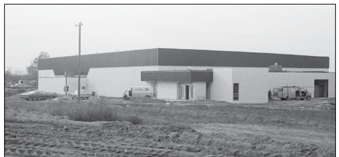
Scugog's new arena under construction in 1976.
