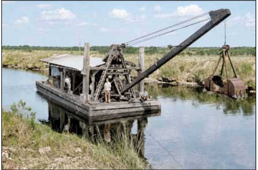
There are no pictures of the actual dredger that carved out the channels in the Scugog Game Preserve, but this photograph of a dredger from the 1920s, provides a concept of the type of machines that may have been used to create 20 miles of canals.
